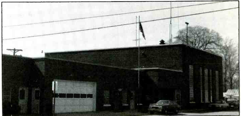
City hall at New Madrid is constructed of masonry. Don't expect much communications from this facility after the quake.
