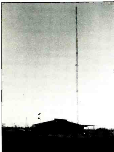
MSHP believes that self-supported towers have a better chance of surviving the earthquake than guyed towers. Hope a trooper is not standing under this guyed tower at the Popular Bluff headquarters when the ground begins to shake.
