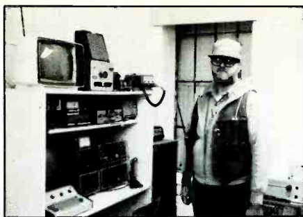
This is the communications area in the Warren County EOC. It is typical of small county EOCs. The equipment is borrowed from local hams and public service agencies.
