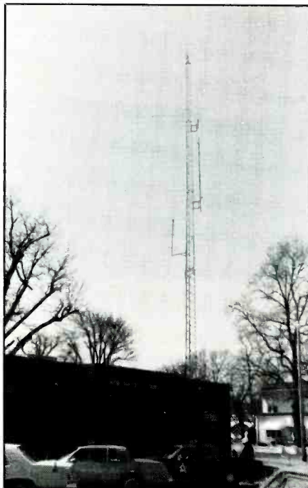
The New Madrid County Sheriff uses a self-supported tower for his communication center.
